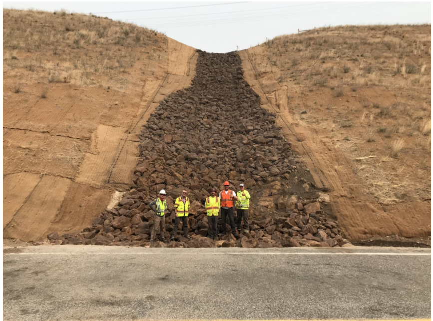
Completed Pebble Beach Repairs
